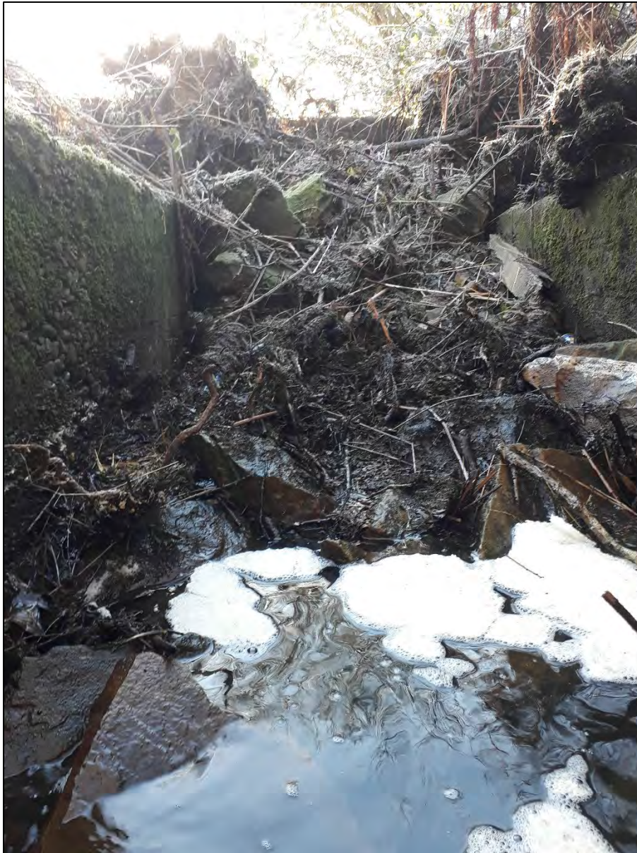
Figure 4.6 Build-up of debris blocking the flow of water in the beck at Walkmill Community Woodland
