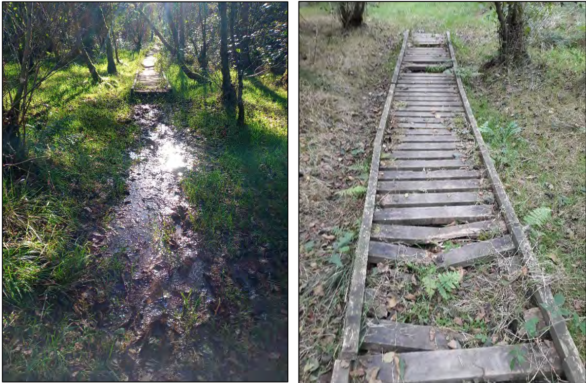
Figure 4.23: Damaged boardwalk and wet, boggy footpath
