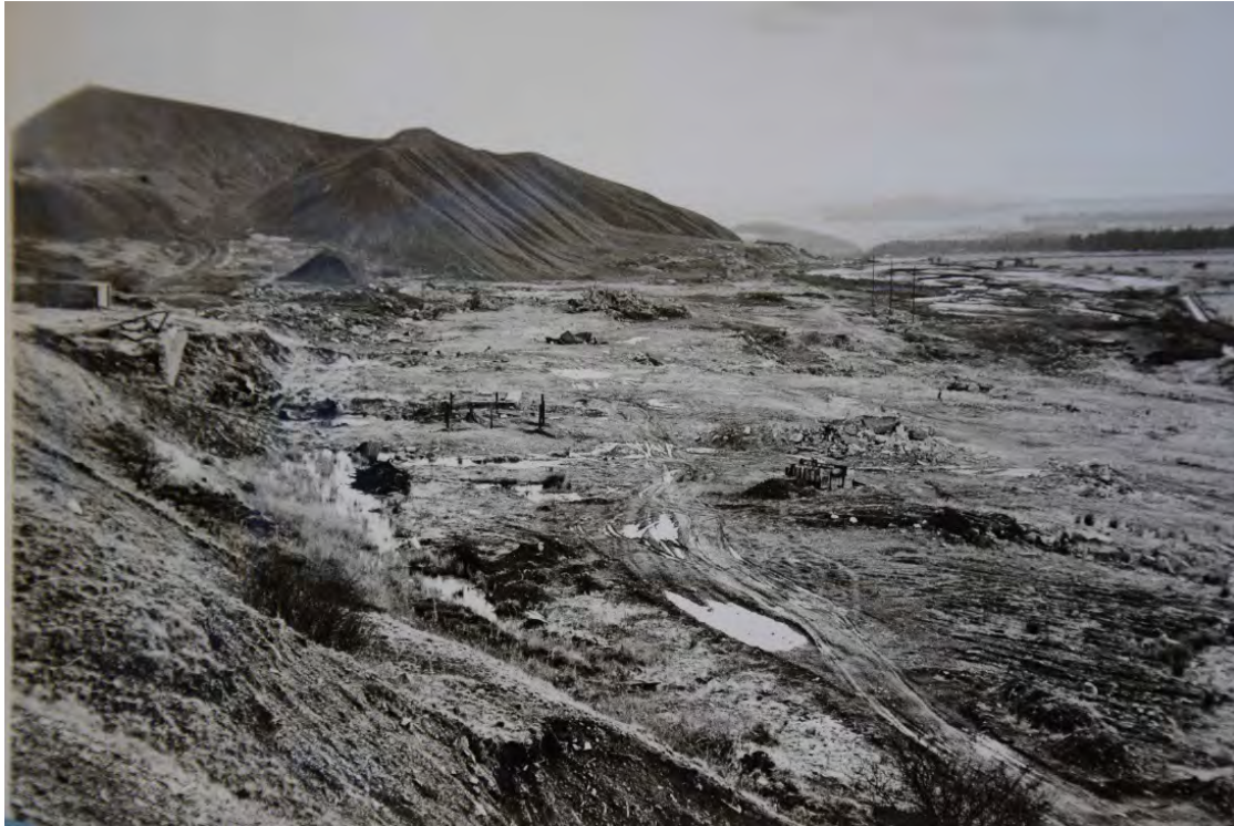
Figure 2.12: A view looking south across the demolished colliery site
