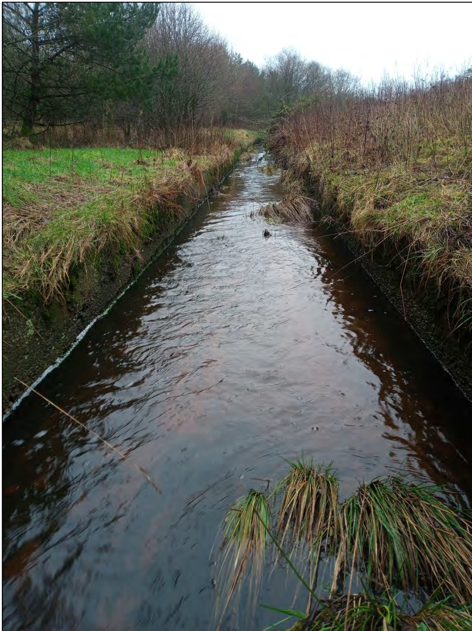
Figure 4.5 Straightened, concrete-lined beck at Walkmill Community Woodland
