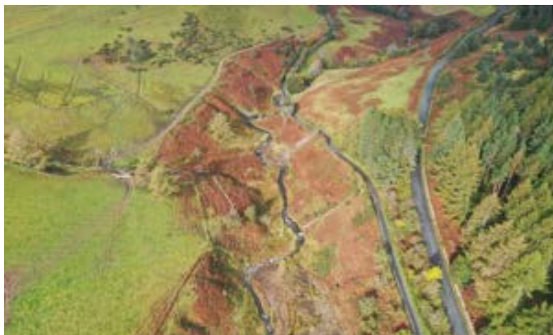
Figure 19: Aerial image of Blaze Beck restoration site, post works.
