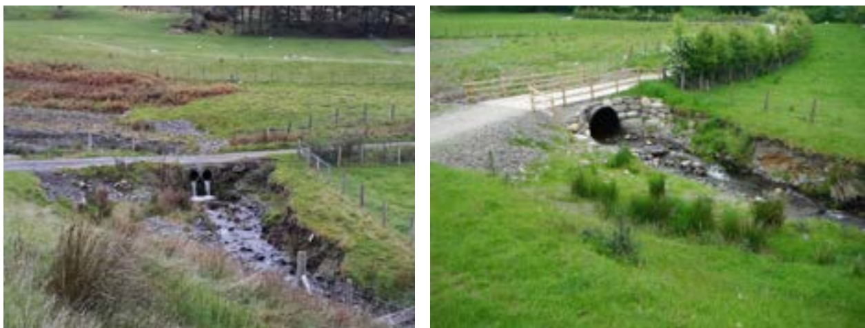
Figure 19: Lonscale culvert upgrade before (left) and after (right) photographs.
